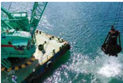
起重機船160t 浚渫
